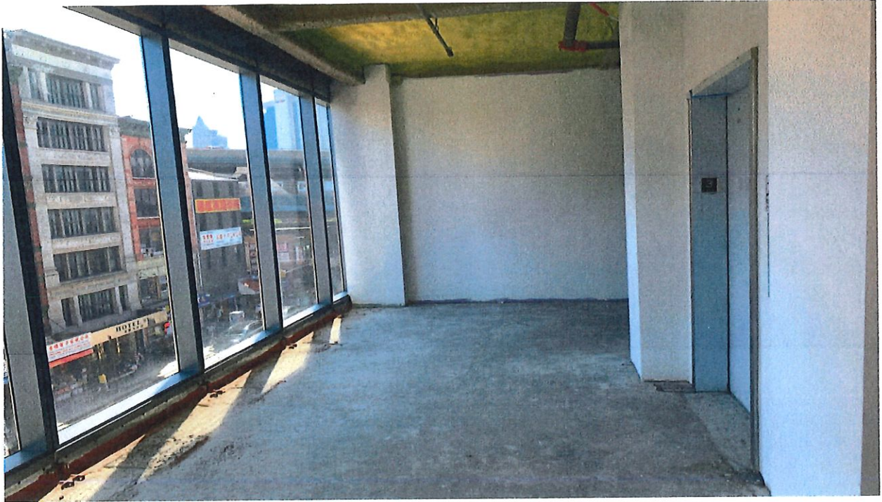
THIRD FLOOR MAIN ROOM
