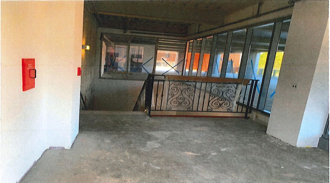
THIRD FLOOR STAIRS
