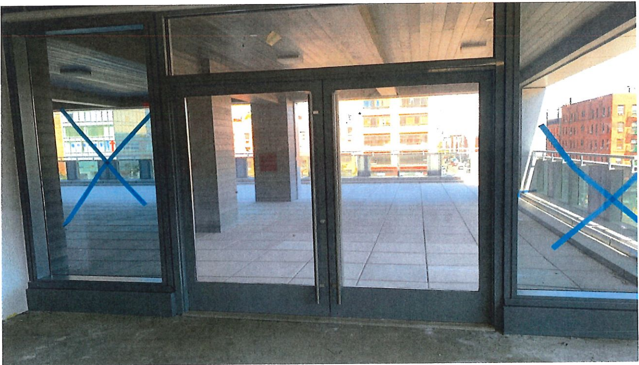
THIRD FLOOR EXIT
